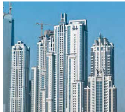
Westbury Tower & Residential Tower, Business Bay, Dubai
