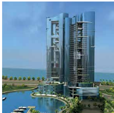
Construction of Saraya Project, Abu Dhabi
