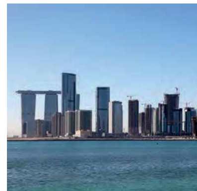
Protection Works of the Marina Square, Al Reem Island, Abu Dhabi
