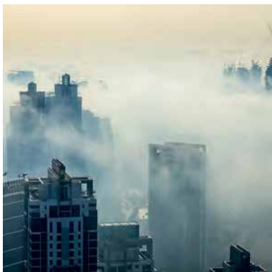
Construction of the National Center of Meteorology and Seismology, Abu Dhabi
