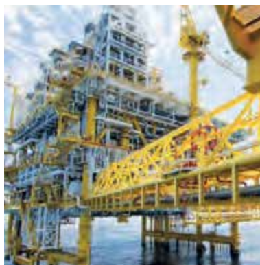
Zakum Development Company EPC Works for Fire & Gas System Upgrade at Zirku, Abu Dhabi
