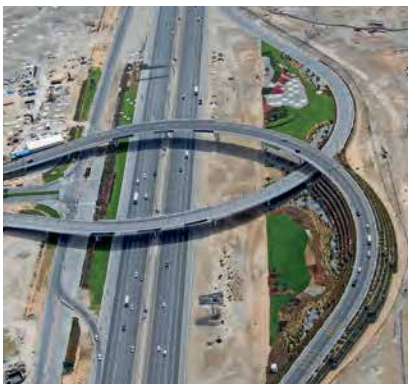
Construction of Dubai Bypass
