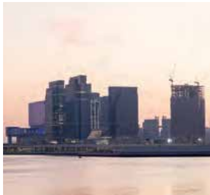
Stock Exchange Fit-Out Works Sowwah Square, Abu Dhabi
